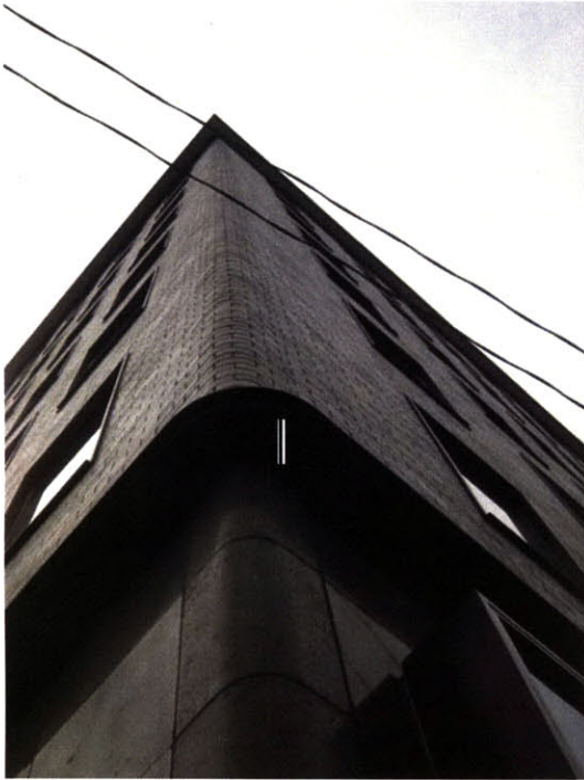
Figure 5.19 Round corner detail of Morigo Building Photograph taken by author.
