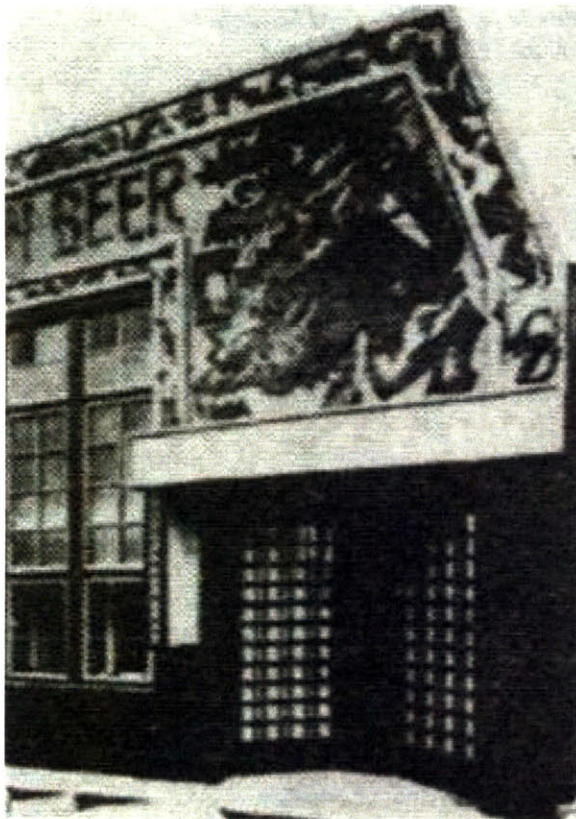
Figure 3.2 Kirin Café (1924) Tokyo - Japan Architect: Barrack Decorating Company Hasegawa, Takashi, Shinden Ka Gokusha Ka - 147
